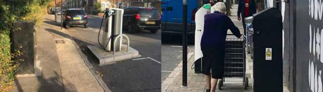
An e-vehicle rapid charge unit located in the carriageway - but note that there will always still be a feeder pillar on the footway.
