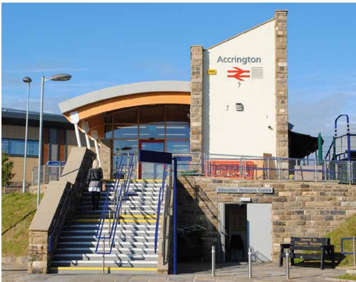
Figure 8 – Accrington Eco station, Lancashire (Image source: Community Rail Lancashire)
