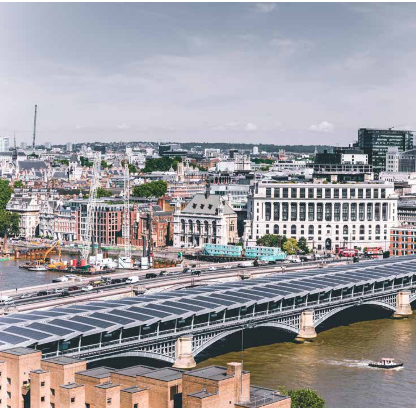
Figure 2 – Blackfriars rail bridge, London
