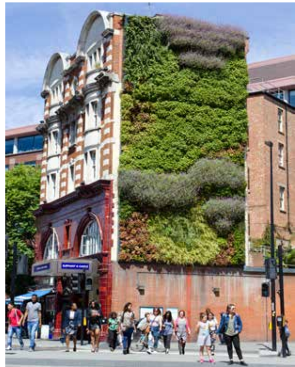
Figure 9 – Green Wall at Elephant and Castle Tube Station, London
