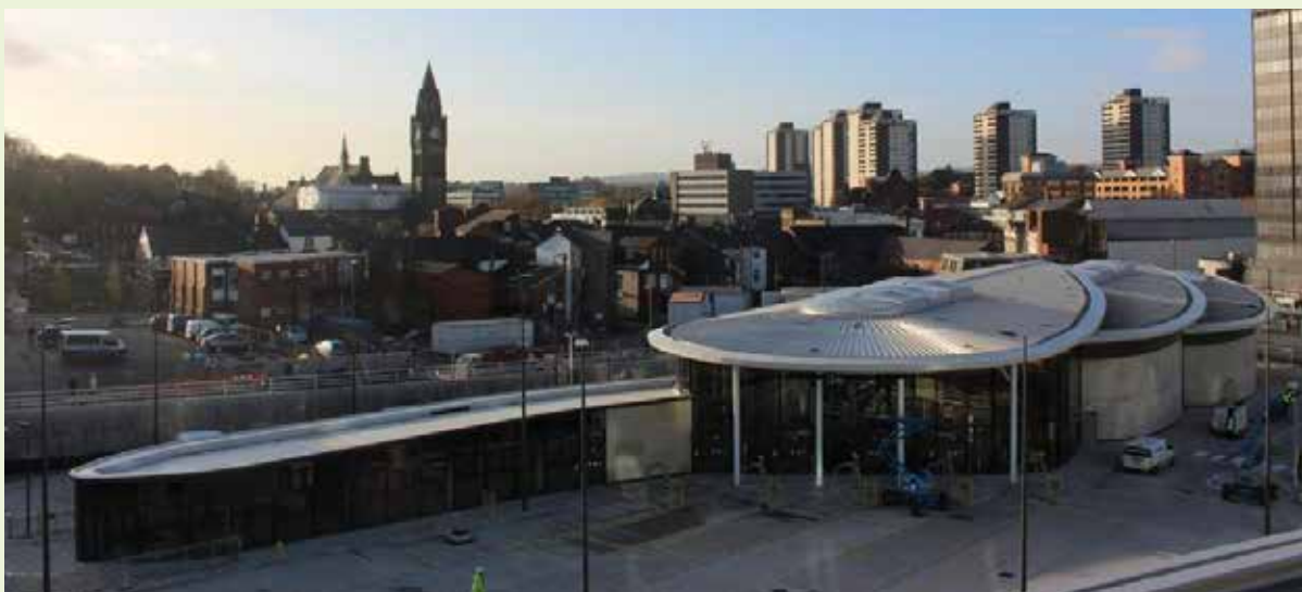
Figure 4 – Rochdale Interchange (Image source: Transport for Greater Manchester)
