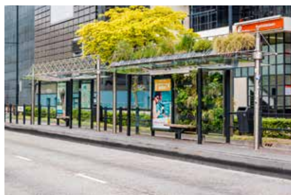
Figure 11 – Green Bus Stop in Eindhoven, The Netherlands
